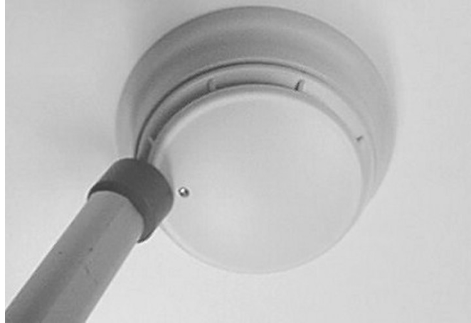
Figure 24. Magnet Test Location for 4098-9601, -9602, -9603, -9605 Smoke Detectors using 553-810 Magnet Tester
